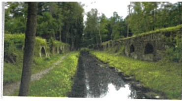
Leetonia Coke Ovens
